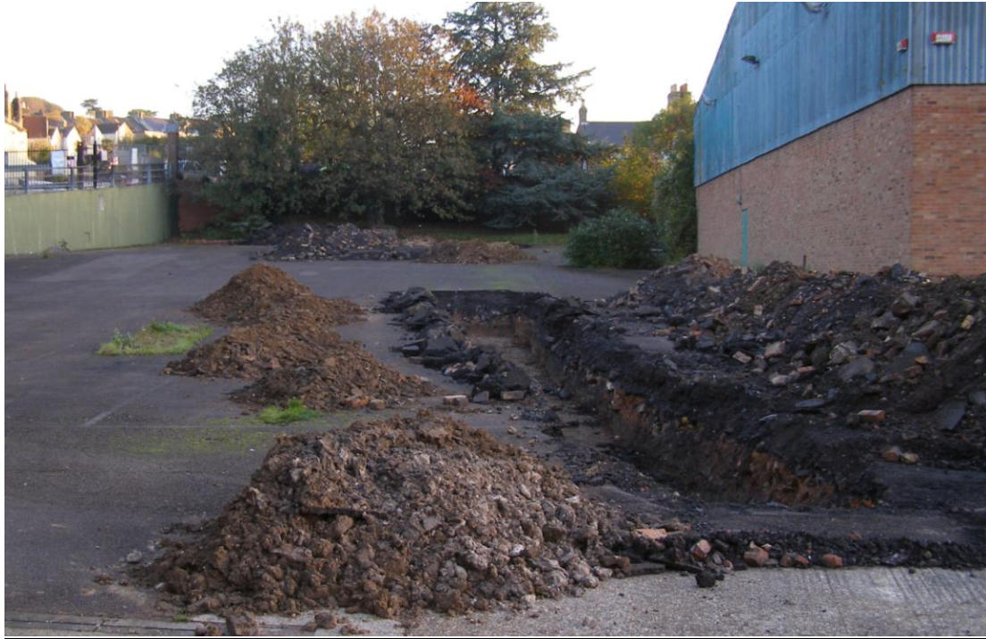
Figure 8: Trenches 1 and 3 (3 in foreground)
